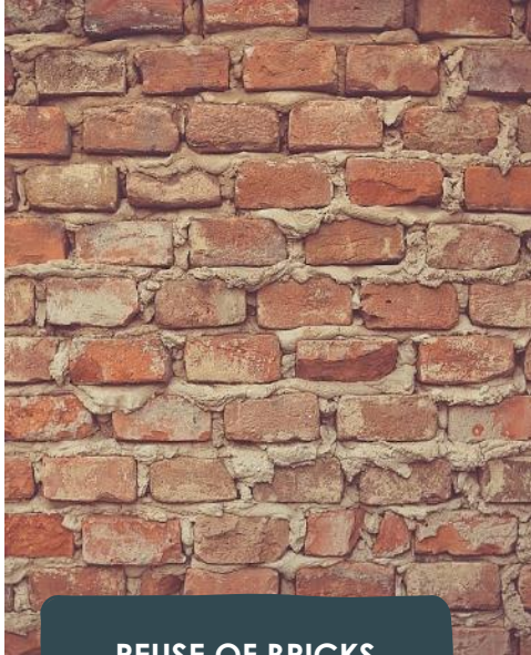
REUSE OF BRICKS
