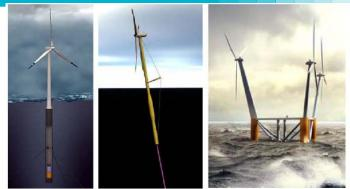
Fig. 1: Floating concepts, from left: HyWind, SWAY and WindSea.
