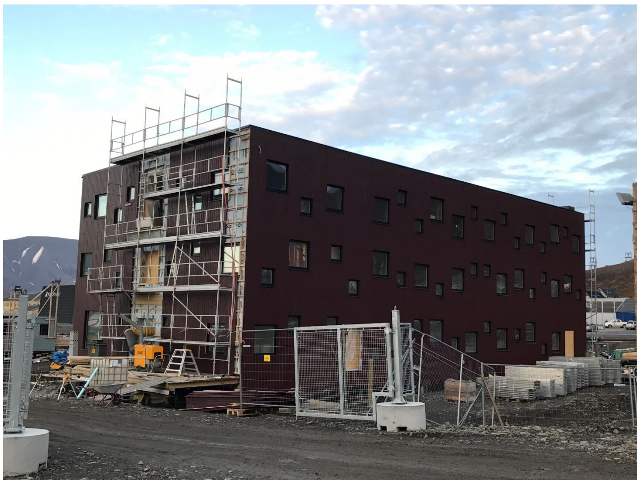
Figure 8. The building "Elvesletta Byggetrinn 1" of a new hotel in Longyearbyen.
