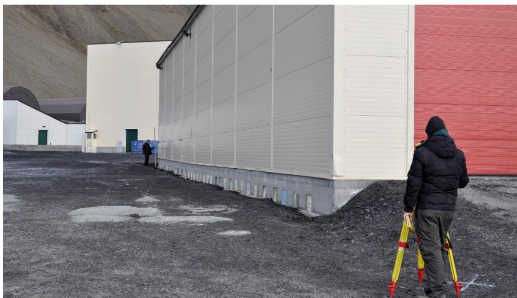
Figure 19. Survey on the multi-purpose garage in Svea.
