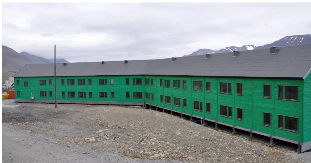
Figure 16. Building of the Låven barakk in Svea.
