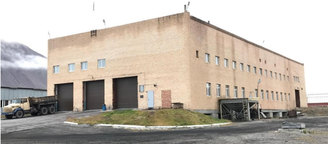
Figure 13. The multi-purpose garage in Pyramiden.
