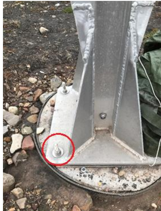
Figure 33. Reference point N4 (PRP4), arrow points on the bolt, on which the bar staff was placed for surveying.
