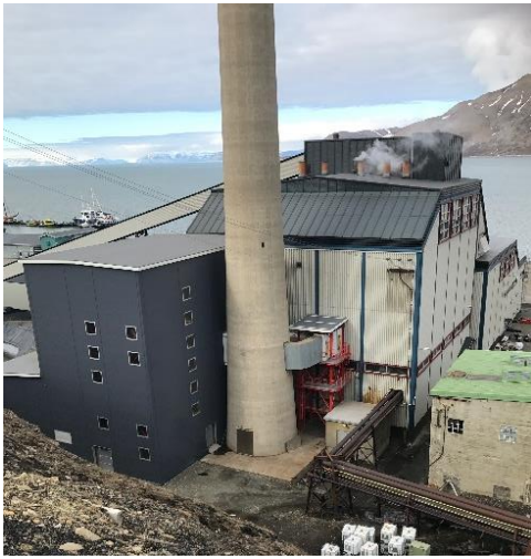
Figure 20. Location of the reference points in Longyearbyen: pipe of the power station.
