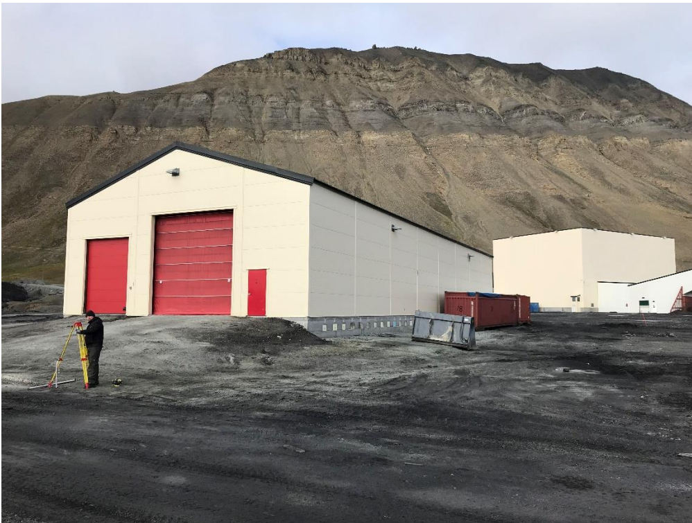
Figure 18. Multi-purpose garage in Svea.
