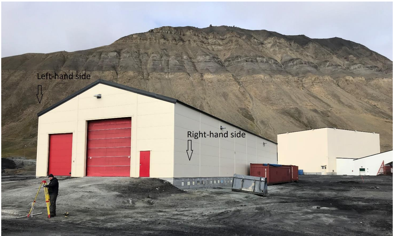
Figure 1. Multi-purpose garage "Magnetittlageret".
